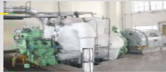
EGG Tesla Turbine 340 kW Runs on waste heat 177°C to 232°C from turbine exh 650 psig + 3 MML/d Desal
