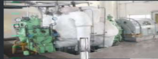
EGG Tesla Turbine 340 kWp Runs on waste heat 177°C to 232°C from exhaust - 650 psig
